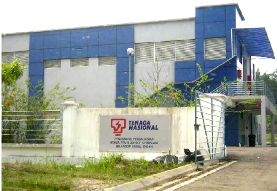
Picture-1: TNB Substation
